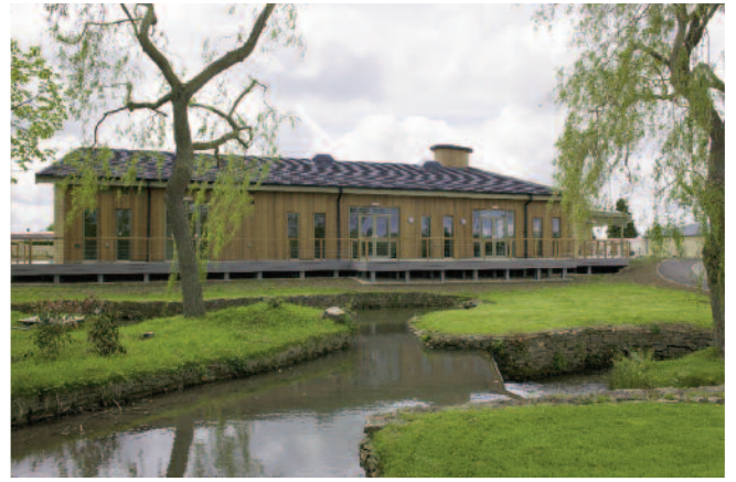
This side view shows how the building sits perfectly into its landscape.
