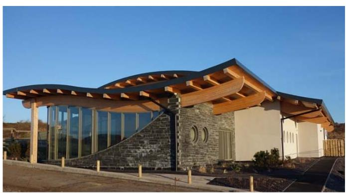
The roof covering is Trocal, in a slate grey colour, which gives the appearance of a seamed lead material. The principal wall construction materials are timber frame supported by glulam timber beams which provide both the vertical wall leg and the curved roof of the structure. All materials are sourced from sustainable sources and are FSC and BM TRADA sourced wherever possible.
